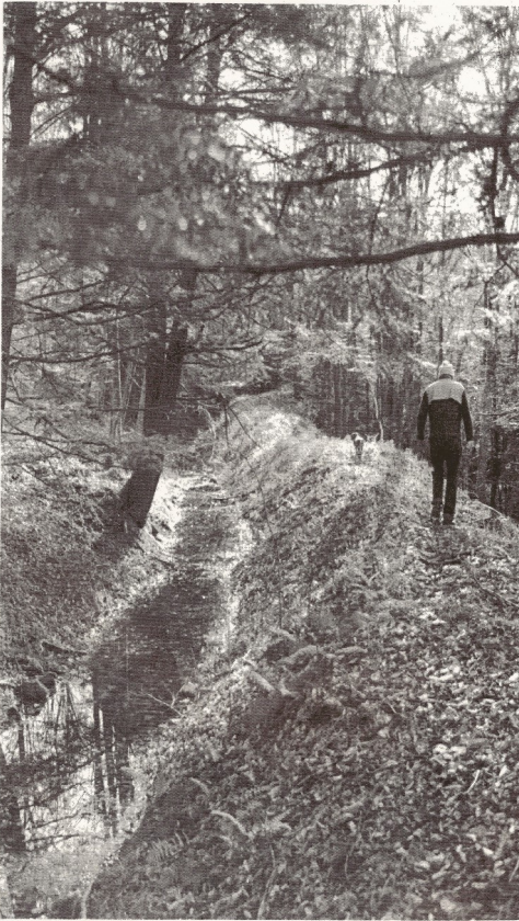
Along the Rock Run - Hunters Lake sluiceway last Sunday afternoon. When Hunters Lake was used to provide power for a hydroelectric generator, and water was in short supply, the trench was opened to supply water from a Rock Run creek impoundment about a mile away. This ditch was dug by hand, pick and shovel and wheel barrow and maybe a horse shovel. Signs are evident that blasting was used here and there.
