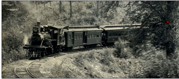
Climbing the mountain at Bully Run curve
